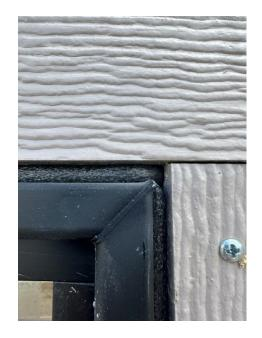
Step 12. Apply a good expandable sealant over backer rod to fill expansion joint and tool it smooth.
