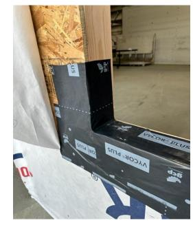
Step 2. Install sill flashing even with the back of the sill and up each side 9" then wrapped down over the top of face flashing.  Step 3. Install shims across sill opening and making sure they are level.
