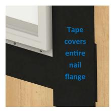
**8)** Apply the head flashing tape in the same fashion. This final section of flashing tape should be the width of the opening plus double the width of the tape, plus 2".
