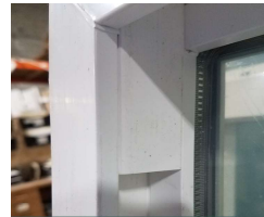
When replacing the sash, be sure to set the sash above the balance shoe
